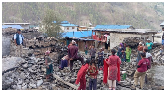
Figure 38: Destroyed houses due to Fire
